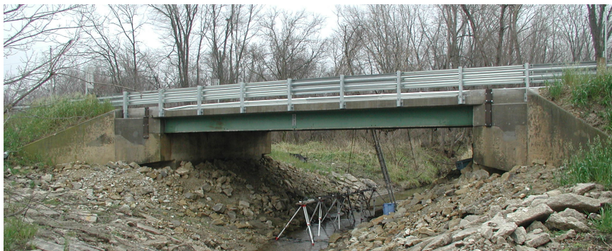
Figure 2.5. Elevation of Tama County SFD bridge.
